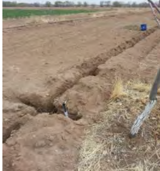
SWCD cooperater installing underground drip.
