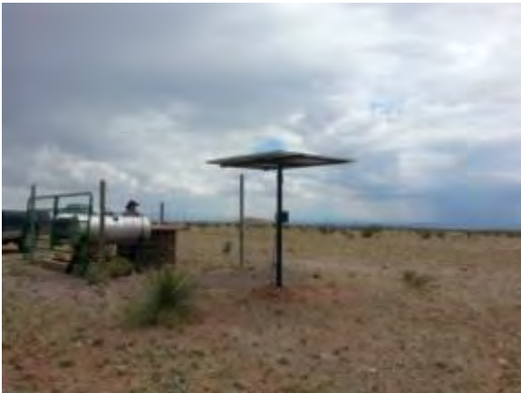
Hickman Ranch diesel to solar conversion, Obsolete diesel pump shown to the left.
