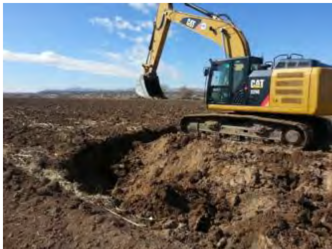
Sub-soiling project underway
