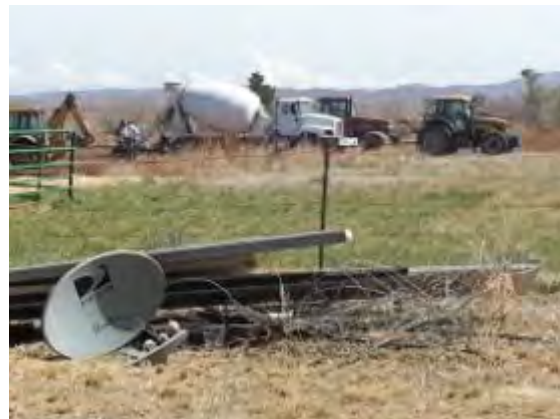
Last portion of ditch being poured.
